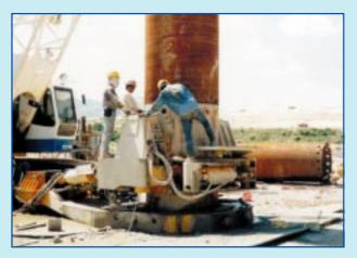
Bored Pile Construction by Oscillator
