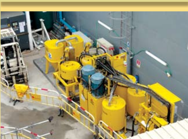
Multi-stage pumping station for grouting of rock shaft in the project
