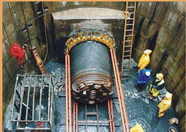
A pipejacking machine suitable for rock excavation is entering a reception shaft through a watertight collar in the UK.
