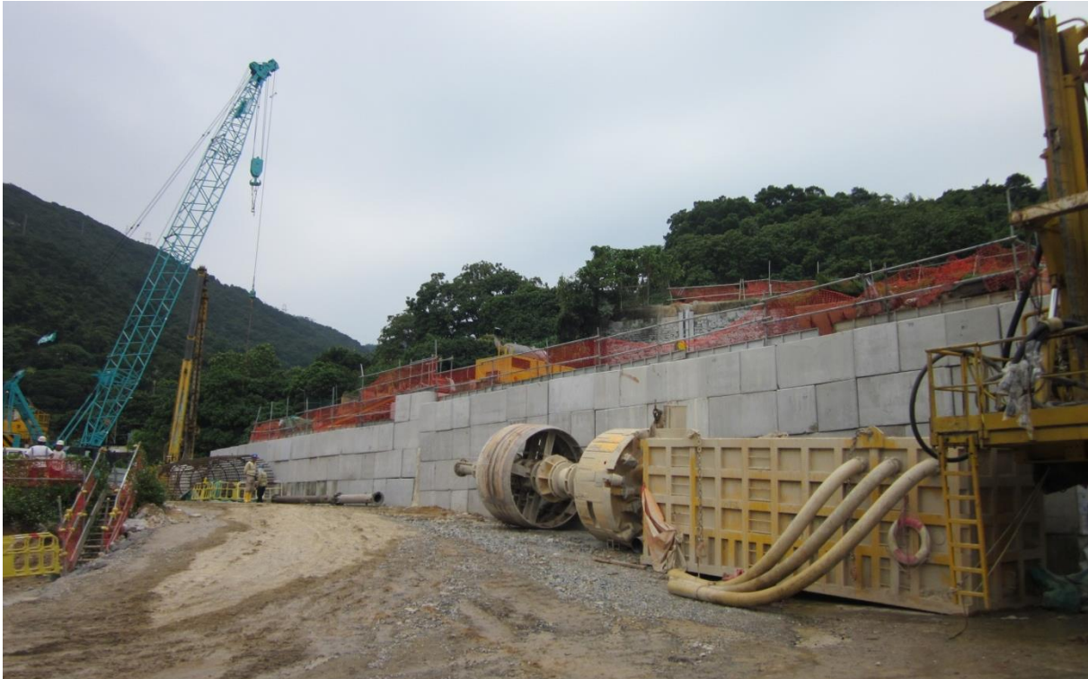
Figure 3 - Traffic ramp and modular block retaining wall
