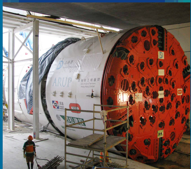
The Tunnel Boring Machine (TBM) was being assembled on site
