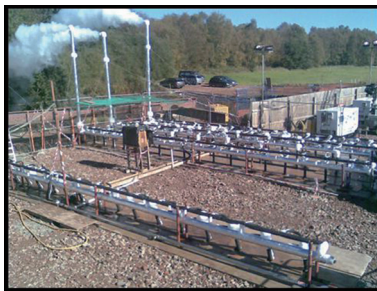
Figure 6 - Ground freezing with liquid nitrogen
