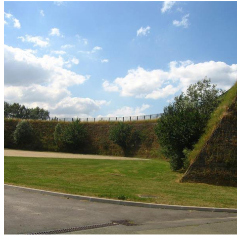
Courneuve park (France)
