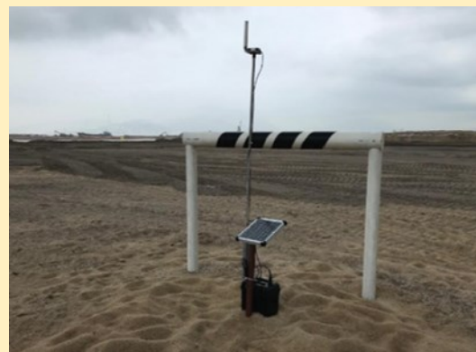
Fig 25 Permanent DGPS Station to Monitor Settlement Marker.
