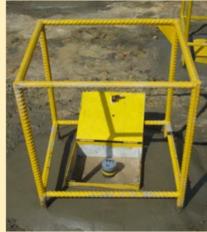
Fig 18 Typical Protection Frame for Instrument on Site Installation/Extension
