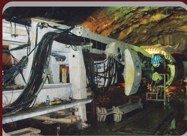
The Robbins 119-222 Tunnel Boring Machine (TBM) was being assembled on site
