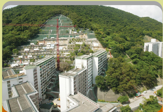
LPM works on slope behind the Sai Wan Estate
