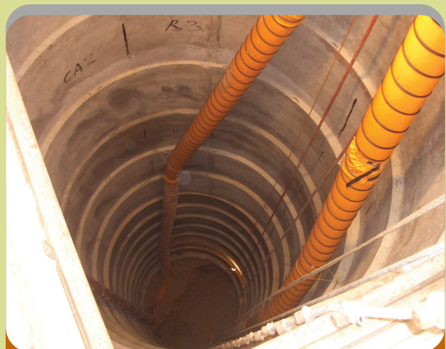
Hand-dug caisson (viewed inside)
