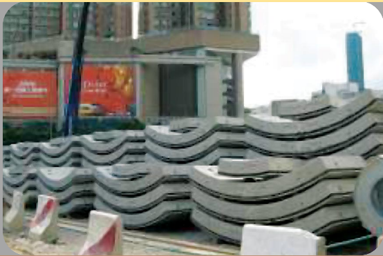
Pre-cast TBM Segments
