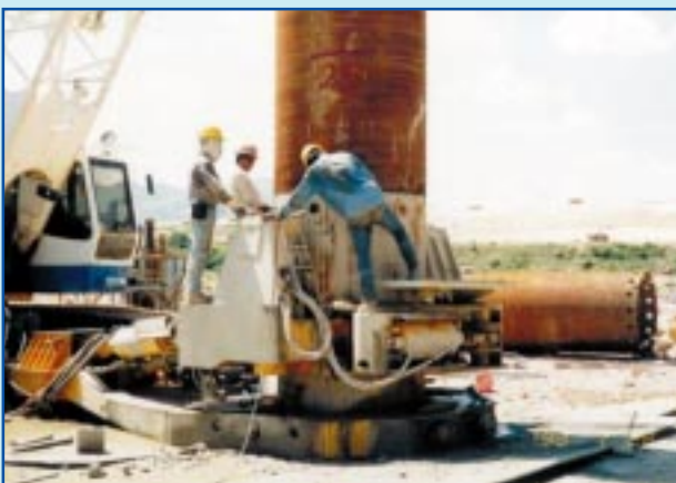
Bored Pile Construction by Oscillator
